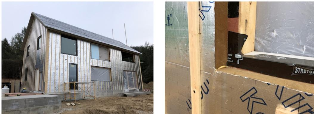
Figure 4. exterior insulation with strapping (left), phenolic foam detail at window opening (pre-flashing) (right).
