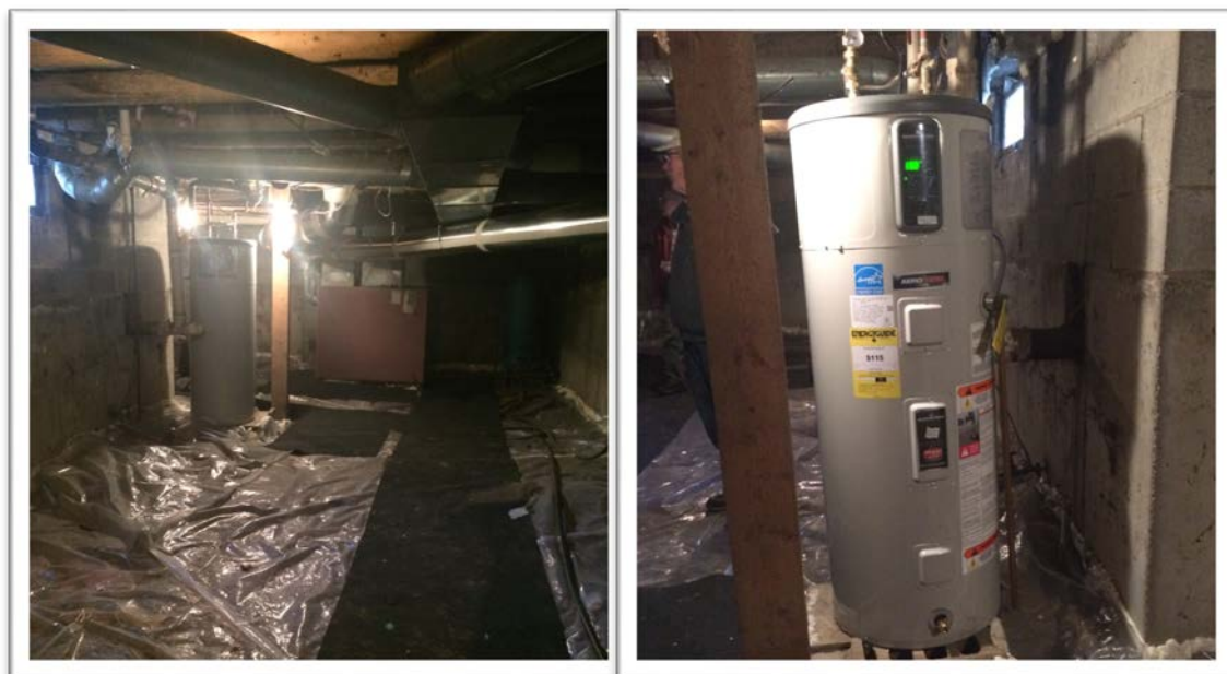
Figure 6. Pilot Home 1 basement encapsulation and repairs.
