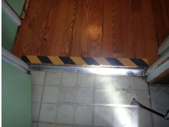
Figure 3: Example threshold with marking to catch the eye and angle added to smooth transition
