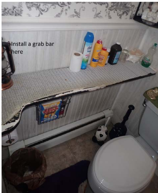
Figure 2: Example photo showing placement of fall prevention measure for installation
