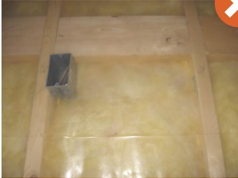
Insulation compressed behind electrical box
