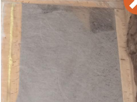
In addition to not having complete fill, the dense-pack fill is not dense enough which means it will settle even more over time
