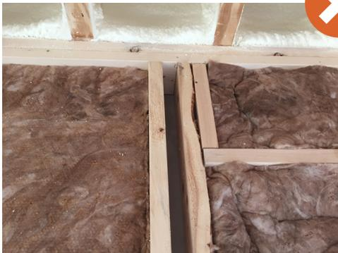
Highly compressed insulation throughout cavity, and missing altogether in some areas
