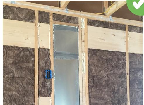
Well-detailed fiberglass, caulk/foam between narrow stud gaps
