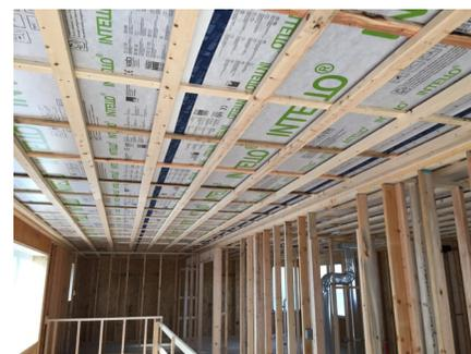
Regardless of where the air barrier is placed, it is important to consider moisture management, vapor control, and the drying potential of the wall.
