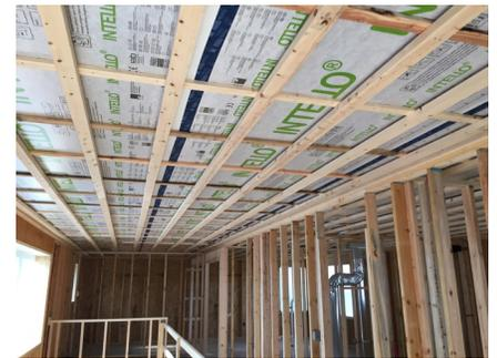
Regardless of where the air barrier is placed, it is important to consider moisture management, vapor control, and the drying potential of the wall.
