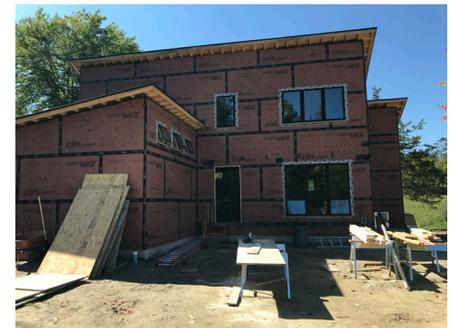
**Limit holes to the exterior.** Consider a condensing gas dryer which does not require venting to the outdoors. Limit, or eliminate, recessed cans in attic/roof ceilings. Relocate the attic hatch access to outside the main living space. Create an access panel through the garage or an attic gable end. Seal all penetrations to the air barrier with a durable, airtight sealant that will last the lifetime of the building.
