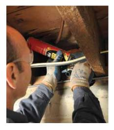
Use low-expanding foam when sealing board insulation against wood rim joints.
