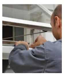
Avoid sealing windows shut with caulk. Use weather stripping on any moving parts.
