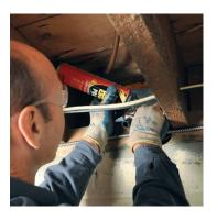
Use low-expanding foam when sealing board insulation against wood rim joints.
