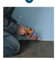
When caulking, hold the gun at a slight angle, and work backward along the seam rather than pushing forward.
