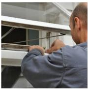
Avoid sealing windows shut with caulk. Use weather stripping on any moving parts.
