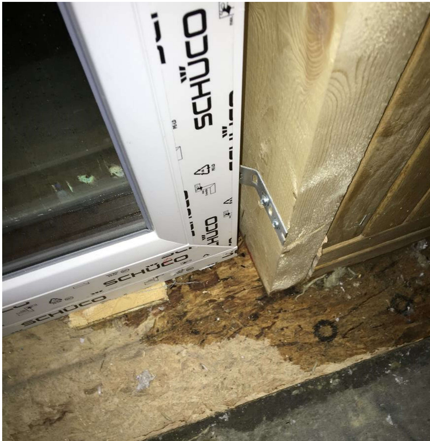
WINDOW SILL- EARLY WATER LEAK!
