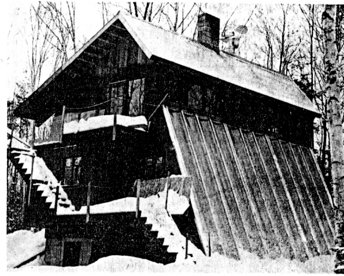
The solar wall on this house in Middlesex collects enough heat on a sunny day even in winter to send inside temperatures to 95 degrees. The steeply angled wall faces south and is designed to collect free heat from the sun to warm Peter O. Hood's home.
