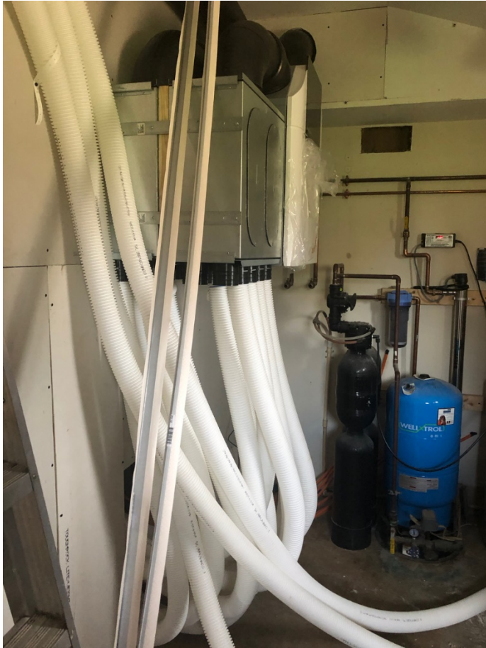
Ventilator hung and initial tubing connections
