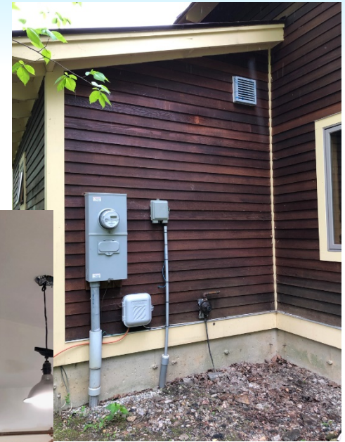
Fresh air intake
