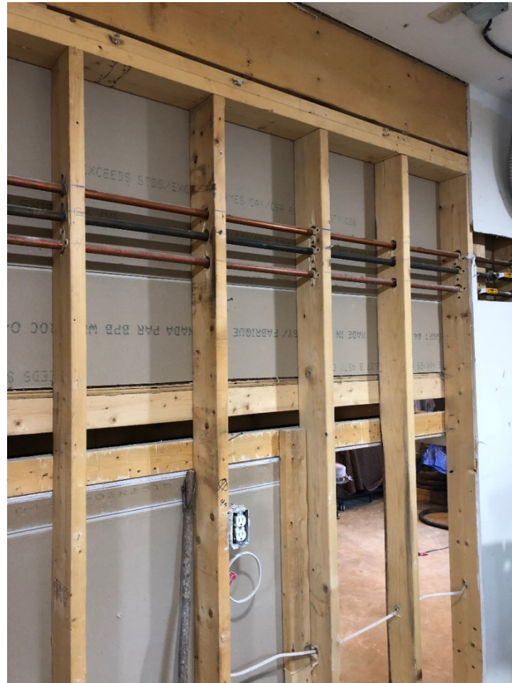
Opening wall to office space
