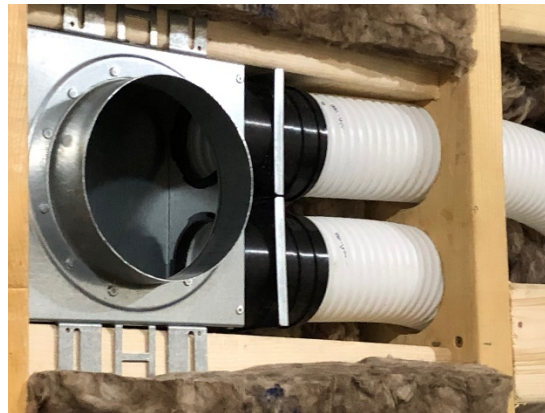
Mechanical room exhaust
