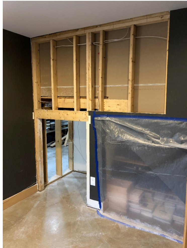
The hope was to stop here... Connection to mech. room
