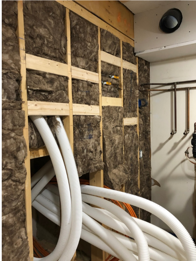
Outdoor air intake
