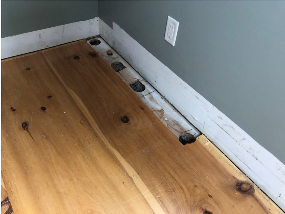
Baseboard out and access for PERT in
