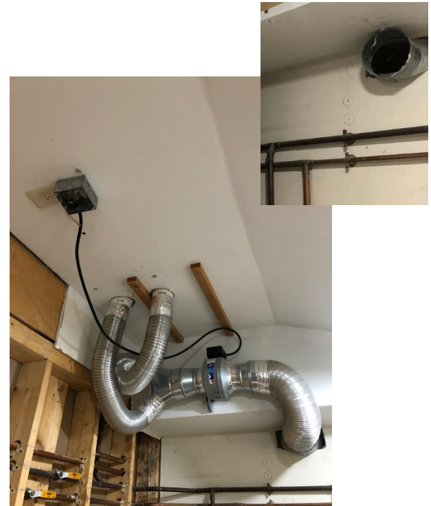
Old exhaust-only ventilation
