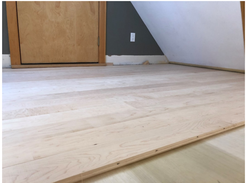
New subfloor and locally-milled maple floor
