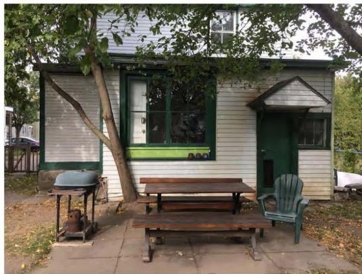
VIEW OF BUILDING FROM BACK YARD
