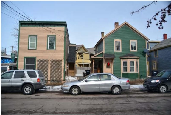
MIX OF FLAT AND GABLE ROOFS
