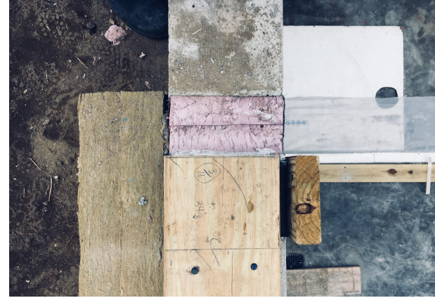
Thermal Break Detail
