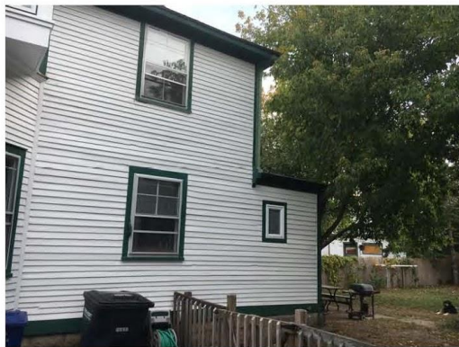
VIEW OF SOUTH WEST ELEVATION FROM DRIVE WAY
