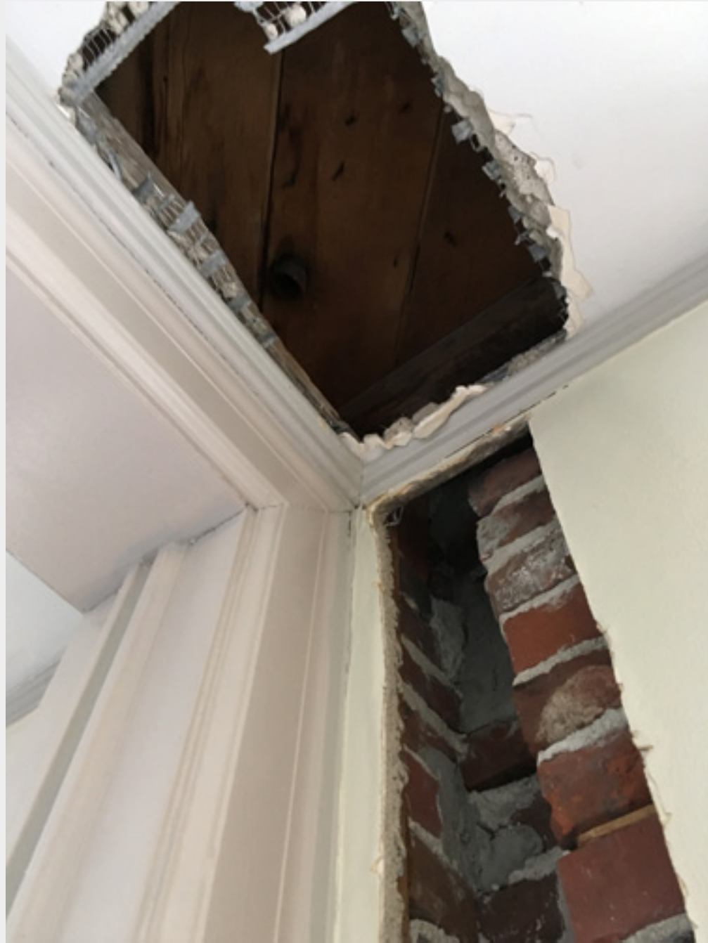
Slade Hall Steam Heat Removed
