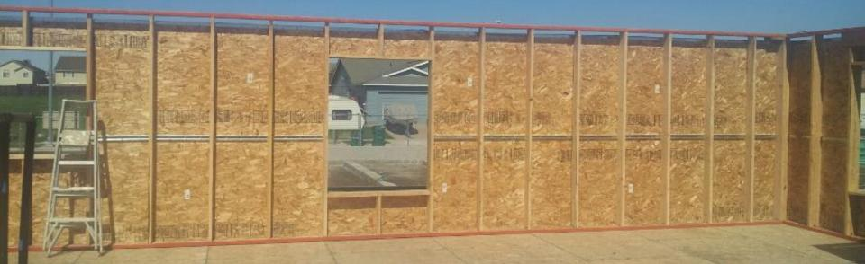
□ 24" OC Single top plates 60-ft LVLs, no lapping needed Windows fit framing (no up-charge for custom size) 35.5% Framing Factor (Sacramento 2014)
