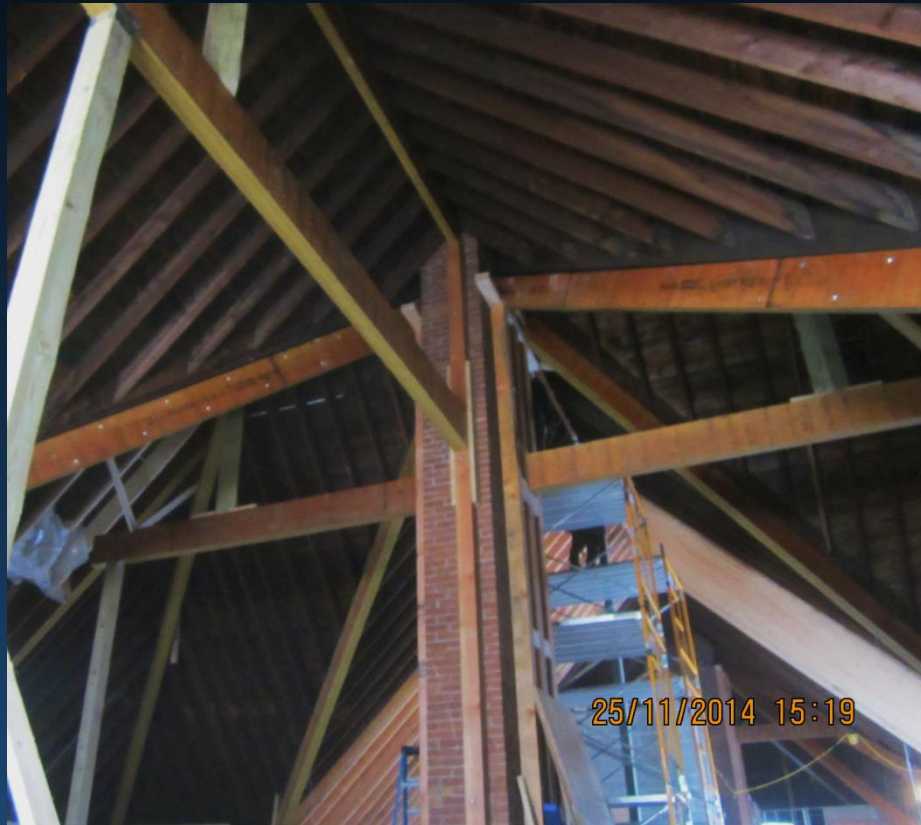
4-PLY 18" DEEP LVL HIP & VALLEY REINFORCING
