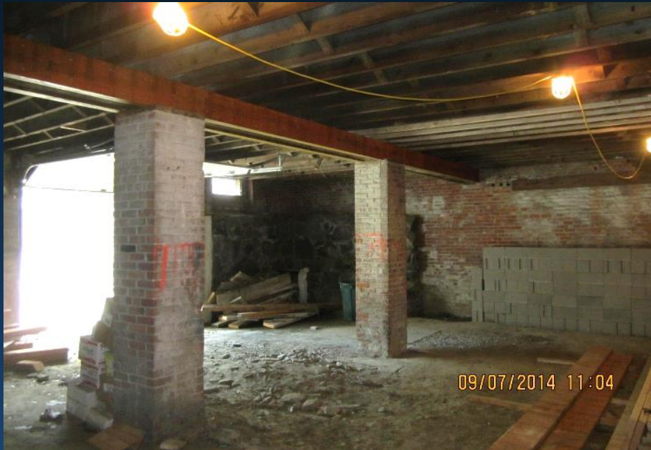
EXSTG FLOOR JOIST SUPPORT w/ (2) 3-PLY 18" DEEP LVL BEAMS
