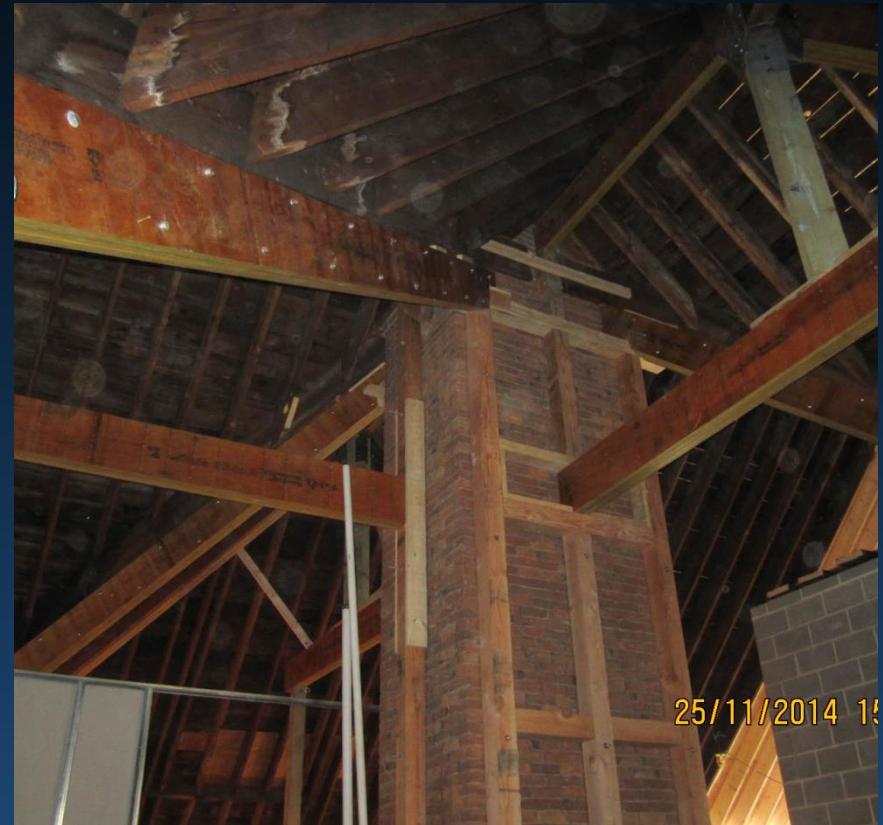
6x6 DOUGLAS FIR REINFORCING @ CHIMNEYS
