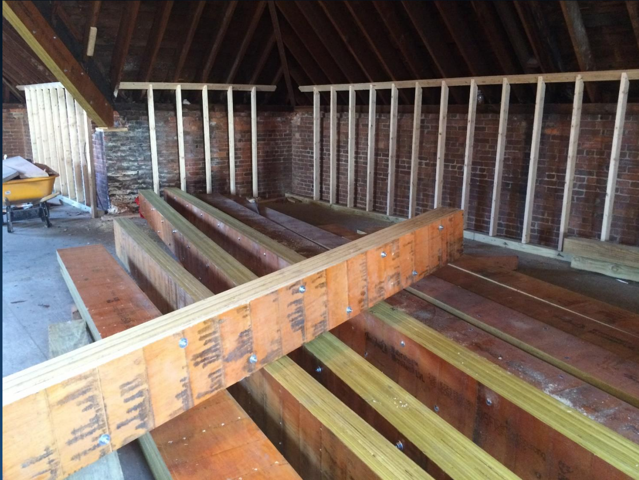
4-PLY 18" DEEP LVL HIP & VALLEY REINFORCING
