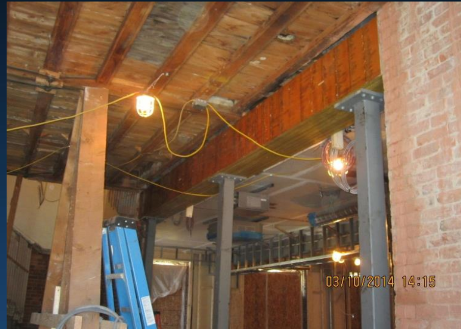
NEW 8-PLY 21" DEEP LVL BEAM @ PRIMARY BEARING WALL
