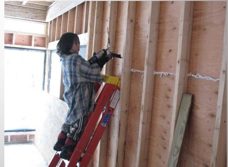
3 – Fixing the leaks
