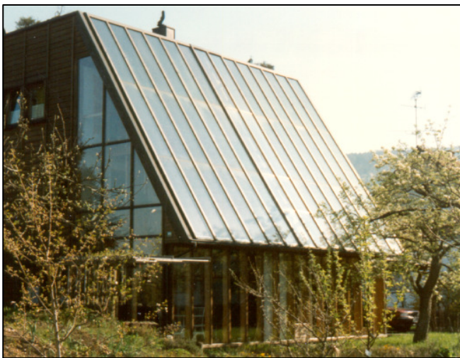
Fig. 6: A solar air collector house Architect: Sture Larsen (AT)
