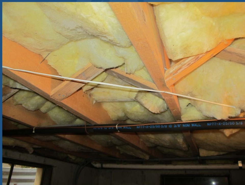
Fiberglass installed in a Cape Cod basement Photo: Alex Wilson
