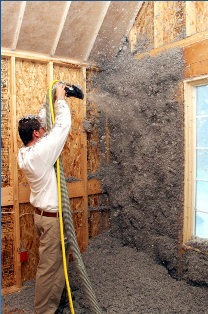
Damp-spray cellulose Photo: EnerSol
