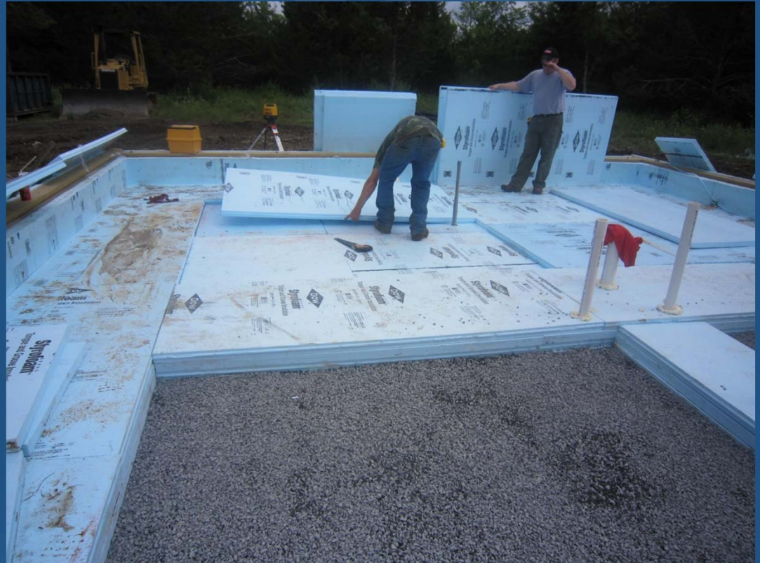
12" of XPS used in passive house foundation— Jordan Dentz photo
