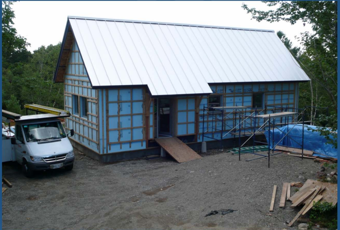
Net-zero-energy house with 4" XPS wrapped around 2x6 walls with cellulose. Photo: Bensonwood
