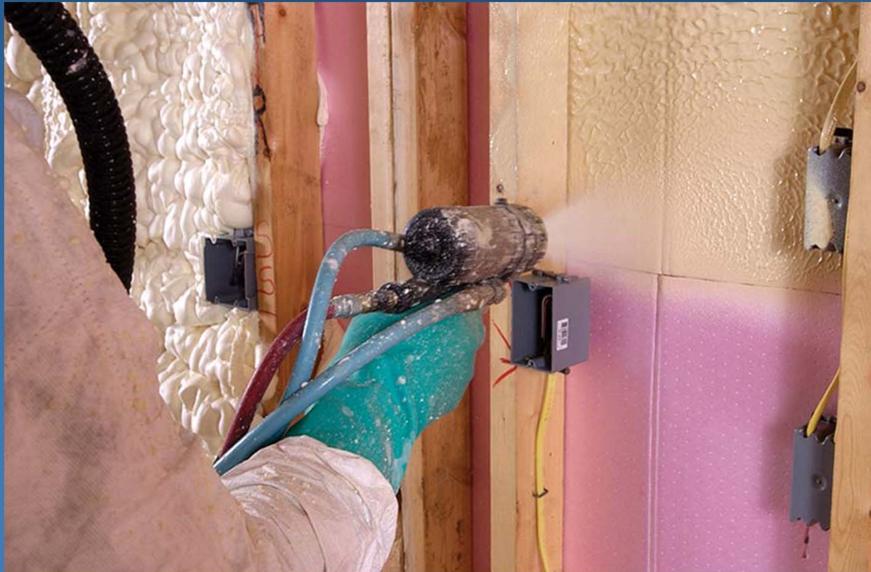
Biobase water-blown SPF - Photo: Biobase
