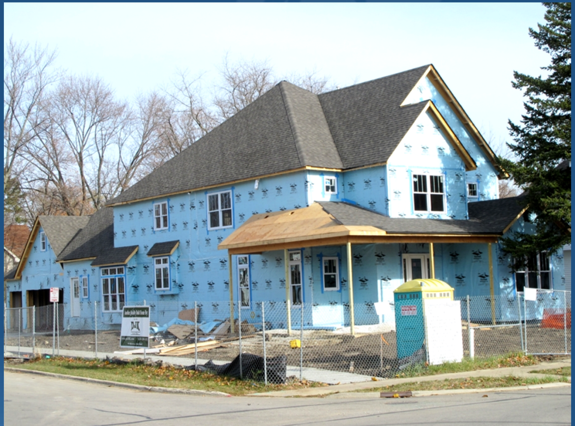
House in Naperville, IL wrapped with XPS Photo: Alex Wilson
