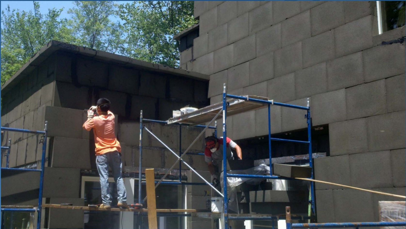
Passive House in Westport, Connecticut insulated with 12" of Foamglas insulation
