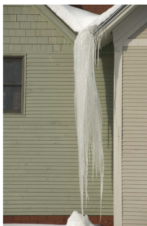
Figure 1: Icicles like this are a good indication of poorly performing insulation and/or ventilation.
