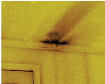
Figure 5: Batt insulation is susceptible to air infiltration. The fiberglass shown here does not stop airflow directly into the home or indirectly into the ceiling section.
