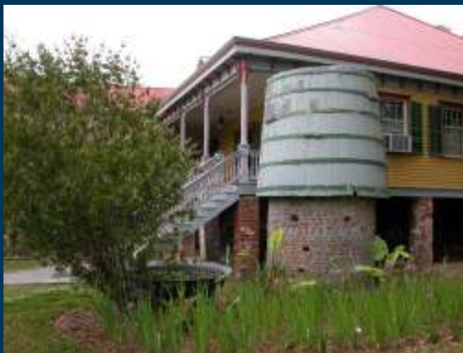
Rainwater cistern - New Orleans
