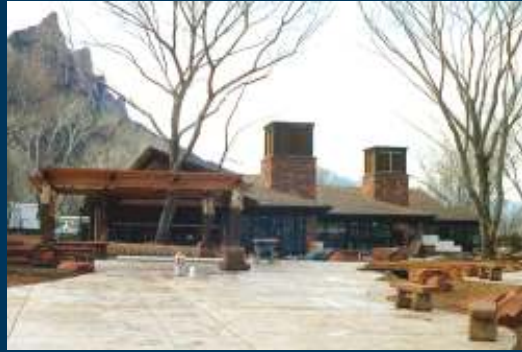
Zion Visitor's Center, Zion National Park showing passive cooling towers in which hot air drawn in at the top and falls down through evaporative pads (NREL photo)
