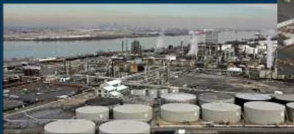
Palsboro, NJ oil refineries, New York Times photo
