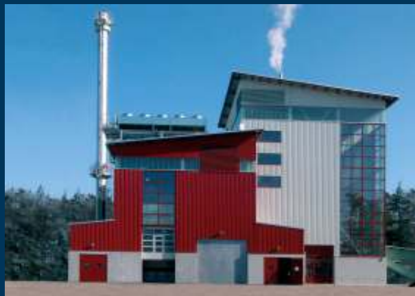
Biomass-fueled combined heat and power plant, Germany Photo: Wärtsilä
