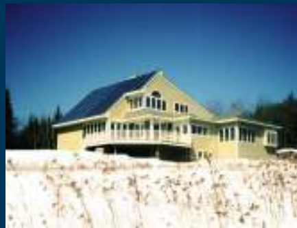
Lord Residence, Maine (Solar Design Associates)
