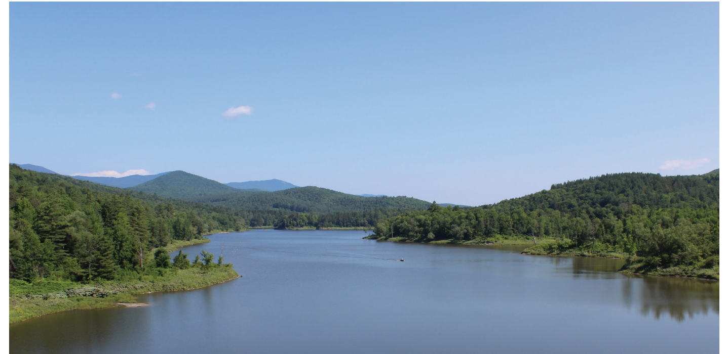
Wrightsville Dam on the North Branch of the Winooski River contributes a portion of Washington Electric Co-op’s 100% renewable portfolio.
