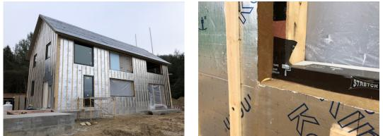
Figure 4. exterior insulation with strapping (left), phenolic foam detail at window opening (pre-flashing) (right).
