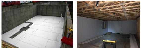
Figure 3. EPS sub-slab insulation (left), polyisocyanurate interior foundation wall insulation (right).
